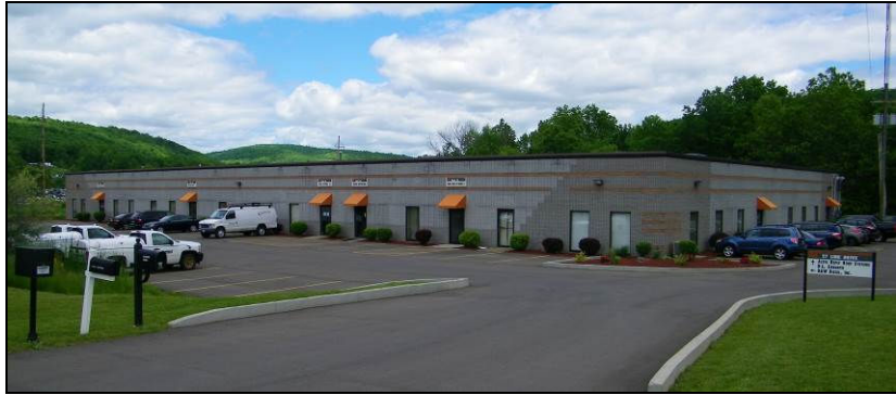
Figure 5 – Western (front) elevation
