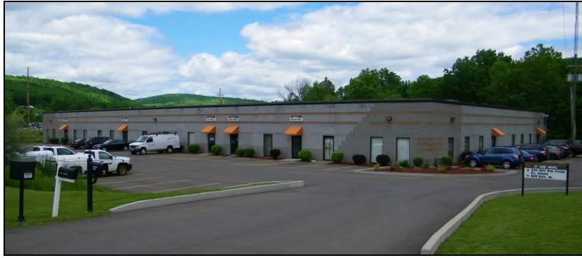
Figure 5 – Western (front) elevation
