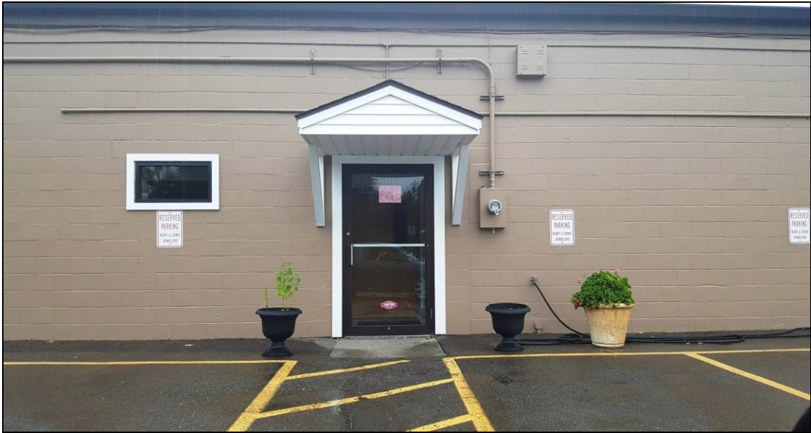
Figure 4 – Entrance of available space
