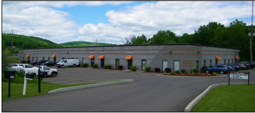
Figure 5 – Western (front) elevation
