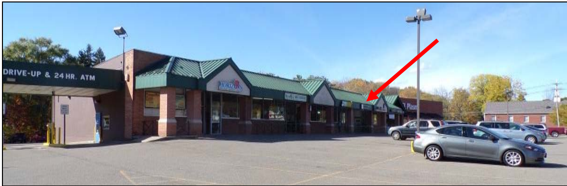
Figure 5 – Front (eastern elevation) of the building
