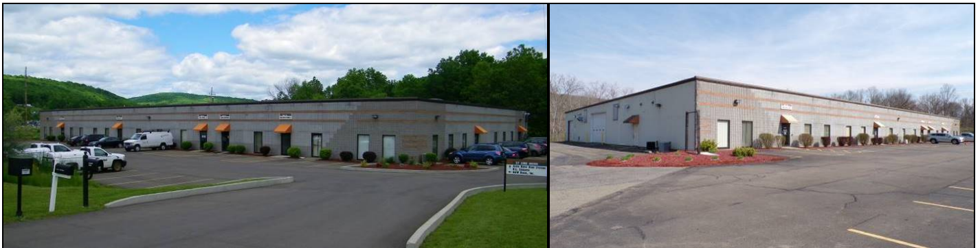
Figure 5 – Western (front) elevation
