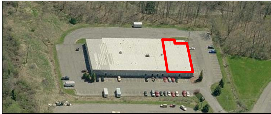
Figure 2 – Western (front) elevation
